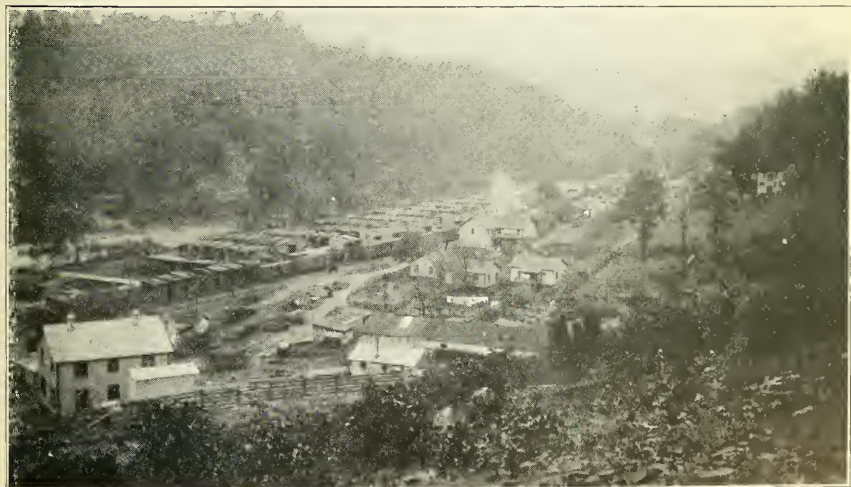
PLATE XXX (b).—Lumber Yard at same plant, with Gauley River at left middle; Topography of Pottsville Series.
